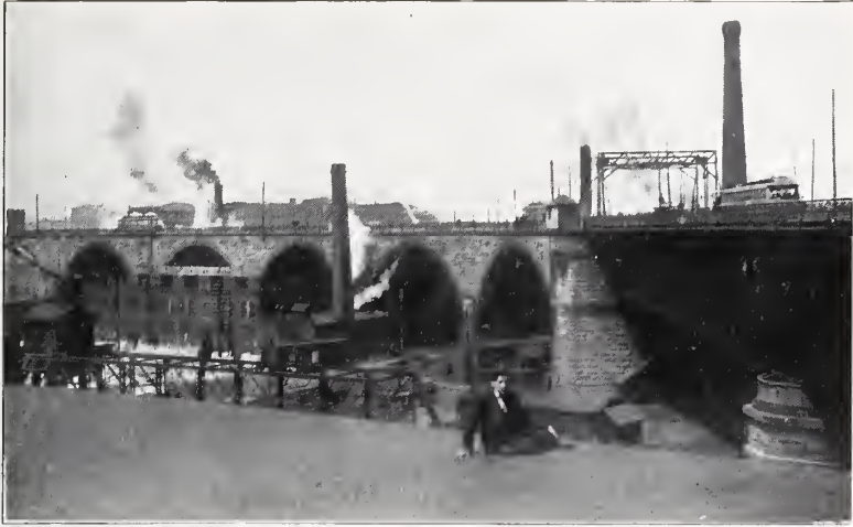
WESTERN PORTION OF THE SUPERIOR STREET VIADUCT, 1909
